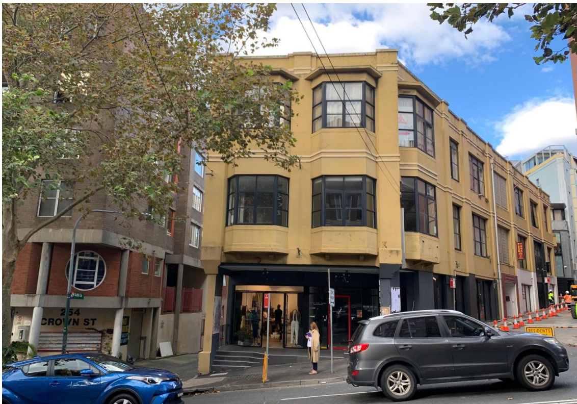
Figure 8: View east from Crown Street towards adjoining mixed use building at 256 Crown Street
