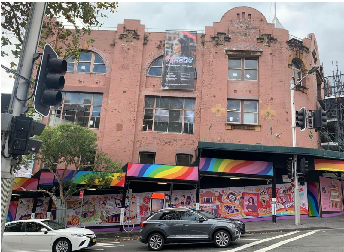
Figure 4: The site viewed from the corner of Crown Street and Oxford Street
