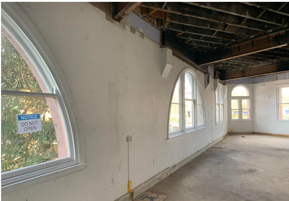
Figure 6: Internal view of level 2 of the subject building looking north-west
