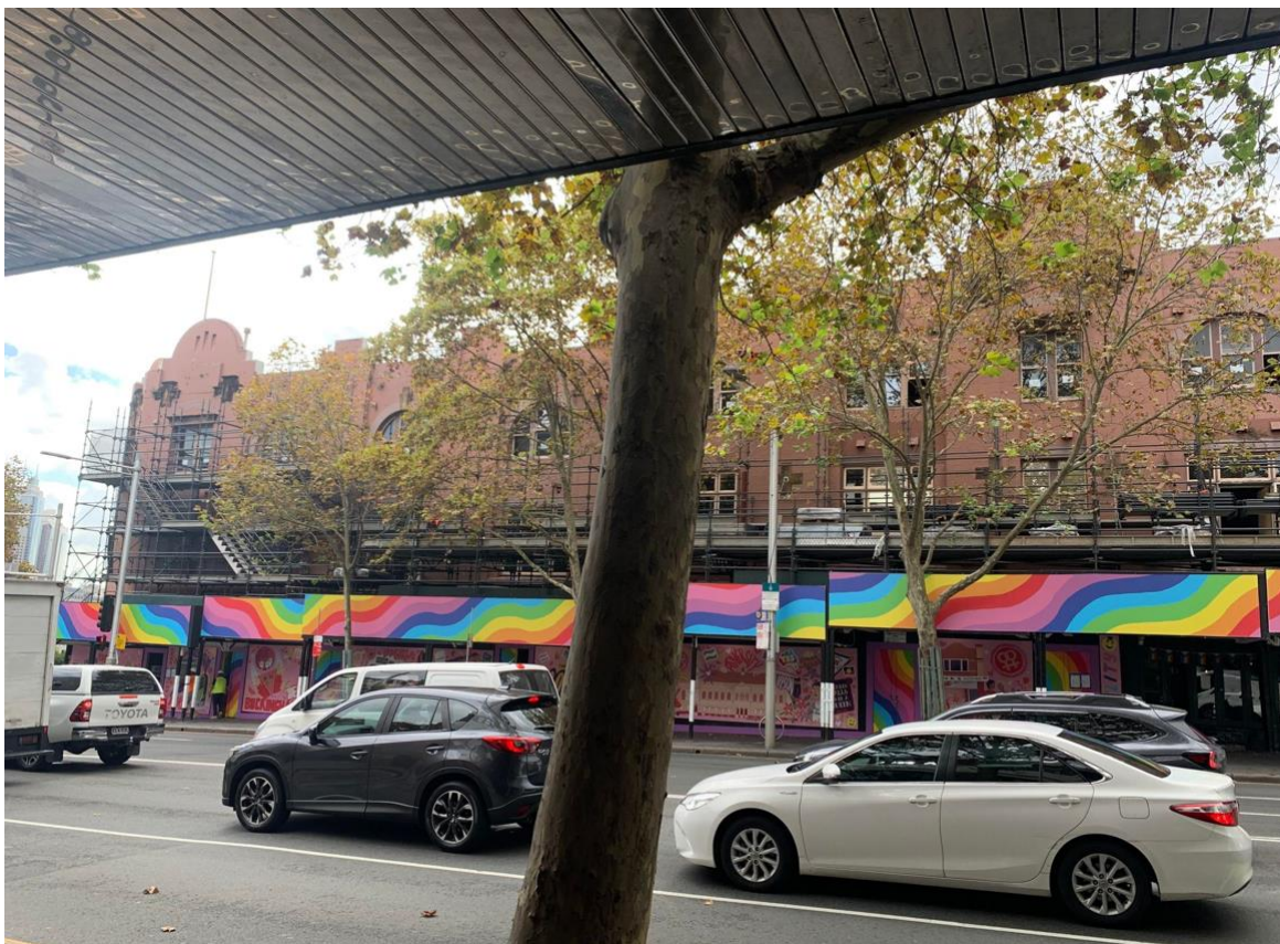
Figure 2: The site viewed from Oxford Street
