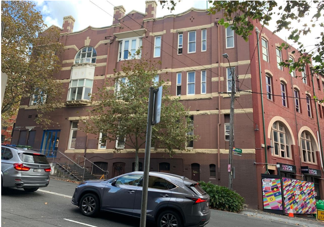
Figure 7: View west across Crown Street towards 80 Oxford Street and Group 1 beyond
