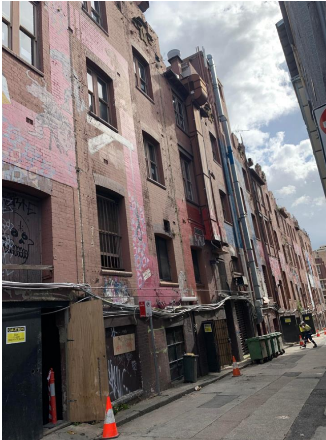
Figure 5: View towards the site from Foley Street
